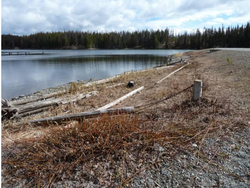
Photo 4.1 U/S Slope of dam – Good condition. Note old log boom.
