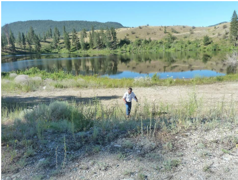
Photo 10.2 From top of dam. Pond elevation is maintained approximately 3 m below top of dam. No emergency spillway.
