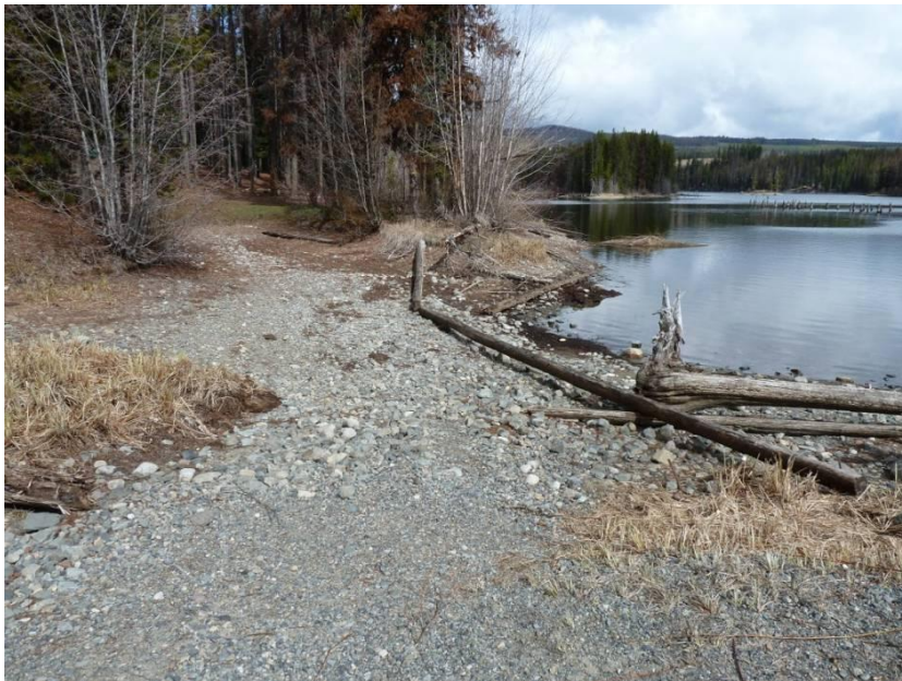
Photo 4.2 Emergency Spillway – Not well defined. Channel requires shaping. Some minor potential for log jams.
