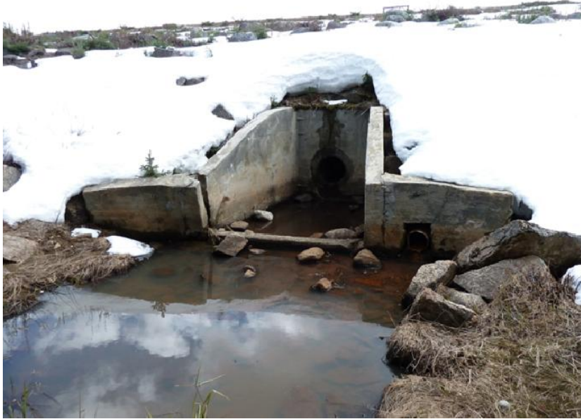
Photo 6.3 Low Level Outlet Structure – Concrete has failed in all directions. Earth sloughing.
