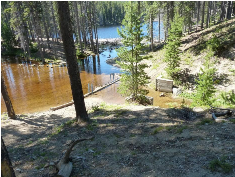
Photo 9.3 Low Level Outlet – concrete in good shape. Some seepage from abutment at structure. Some flow. Note water, but no flow from outlet.
