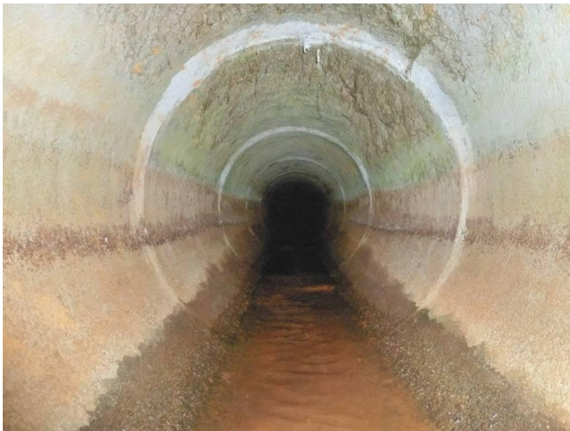
Photo 4.4. General Note: Concrete Conduit in good condition.
