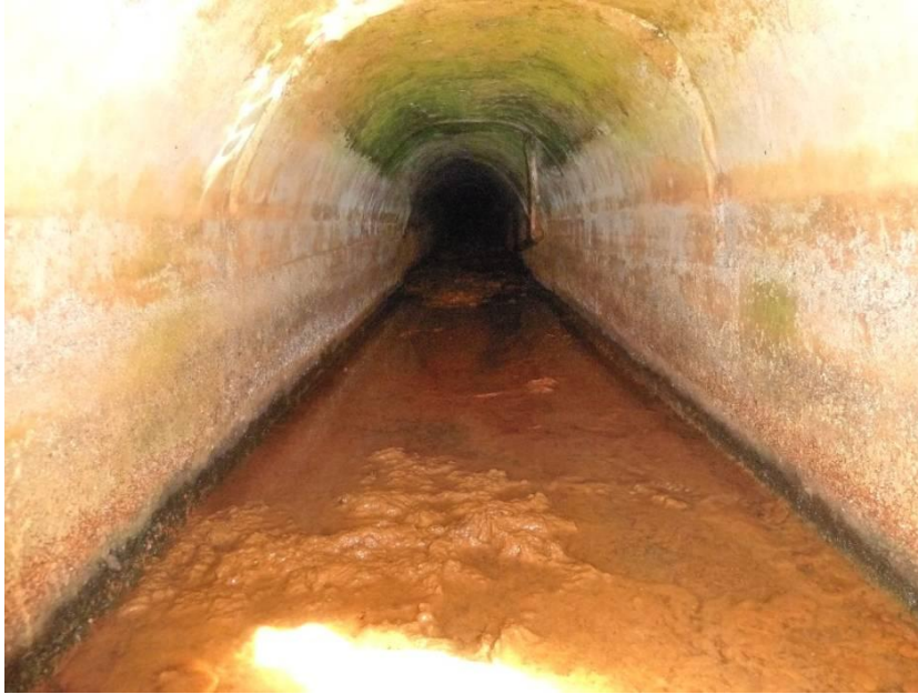
Photo 3.3 Low Level Outlet Structure – parabolic channel in good condition. Requires more frequent exercise to clear dirt and debris.
