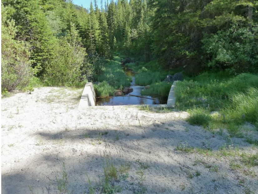
Photo 9.3 Low Level Outlet – concrete in good shape. Some seepage from abutment at structure. Some flow. Note water, but no flow from outlet.
