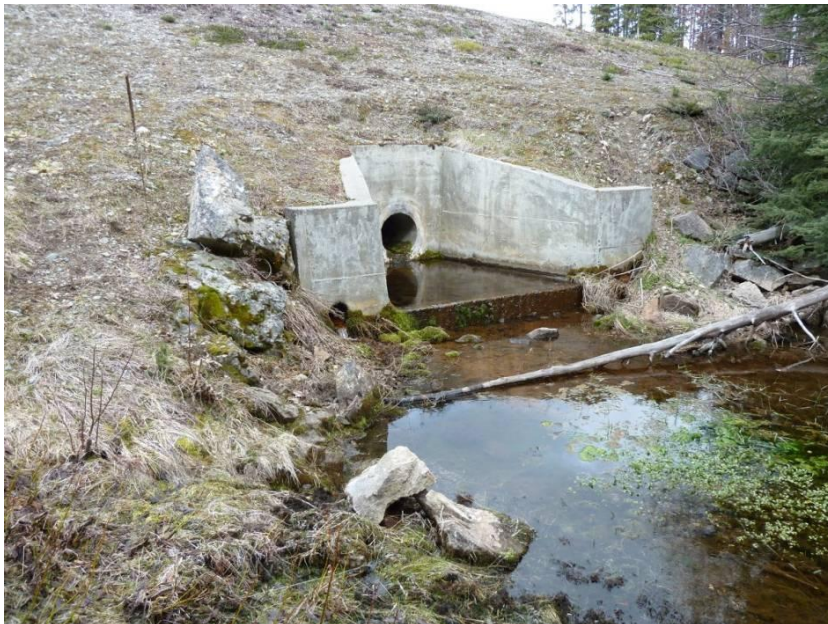
Photo 2.3 Low Level Outlet Structure – Deflection in outlet of CSP pipe. Monitor for further deflections or failure. Requires more frequent exercise to clear dirt and debris.
