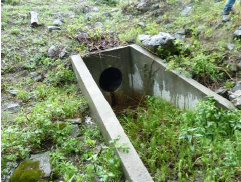
Photo 7.3 Low Level Outlet – concrete in good shape. Backfill and riprap require maintenance around structure. Some earth sloughing. Clean out of debris required.
