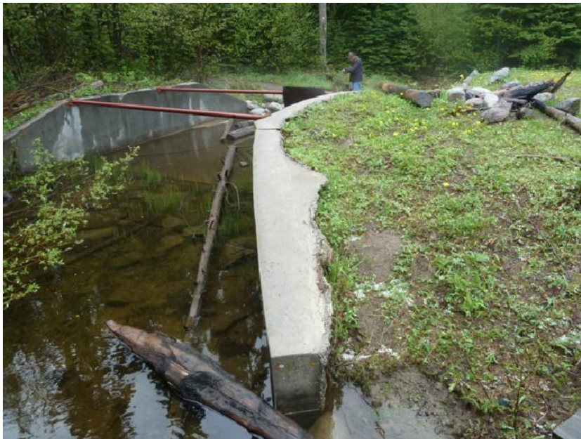
Photo 7.2 Emergency Spillway. Significant earth slouging and lack of riprap on both sides of vertical walls. Concrete failed in several locations.
