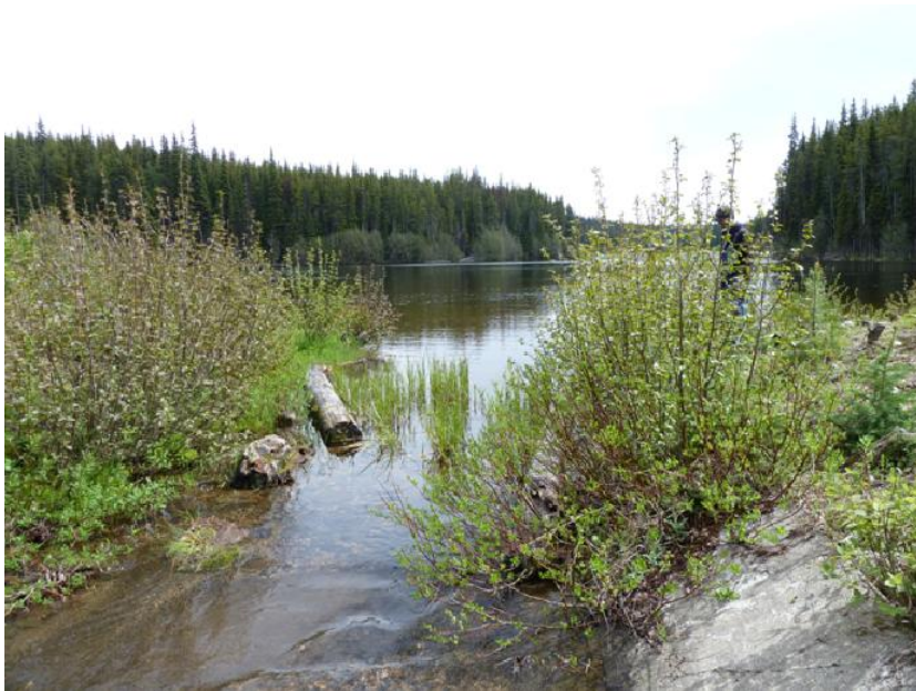
Photo 8.2 Emergency Spillway. Channel through dam. Minor brush removal required. (Performed during site visit). Note concrete entrance. No log boom.
