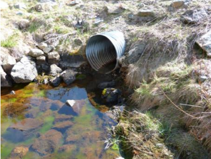
Photo 1.3. Low Level Outlet Structure
