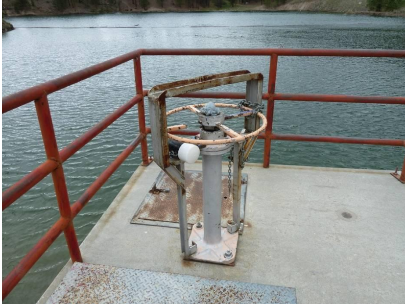
Photo 11.5 Low Level Outlet – Handwheel requires replacement.
