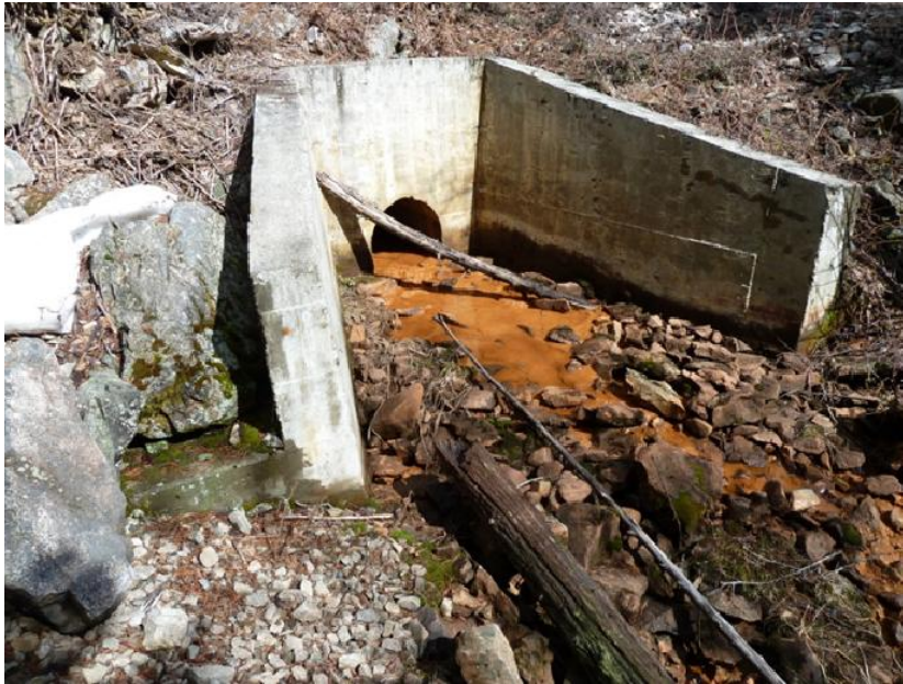
Photo 3.1 Low Level Outlet – Backfill and replacement of riprap required around structure. Rocks, debris and dirt clog outlet.
