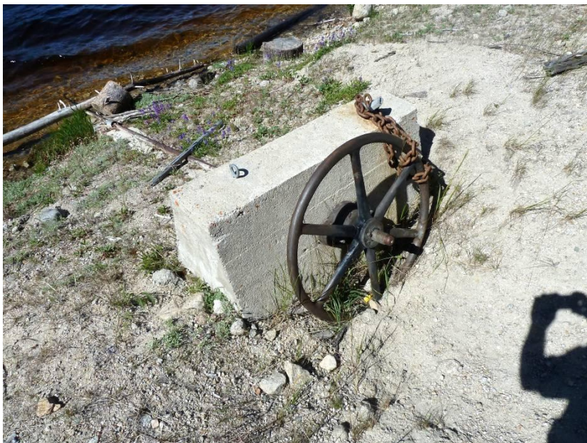
Photo 9.2 Low Level Outlet gate – Adjustment of backfill required to operate gate.
