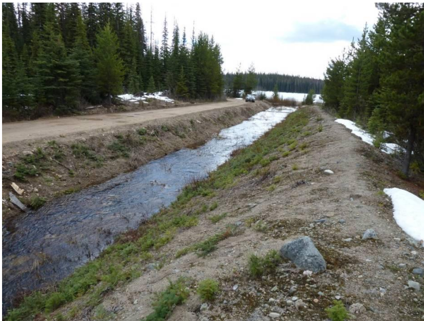
Photo 6.2 Emergency Spillway Channel – Operational. Channel maintenance and cleaning required on a regular basis.
