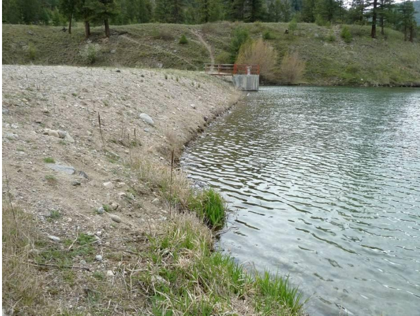
Photo 11.1 U/S Embankment – 1:1 slope, no riprap. Some erosion at base.
