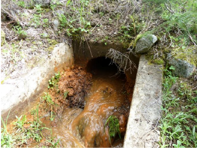
Photo 8.3 Low Level Outlet – concrete in good shape. Backfill and riprap require maintenance around structure. Some earth sloughing. Maintenance was performed during inspection.
