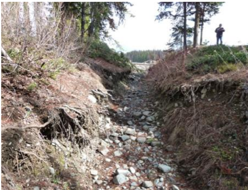
Photo 3.2 Emergency Spillway – Signs of significant use. Channel requires shaping. Potential for log jam is high.
