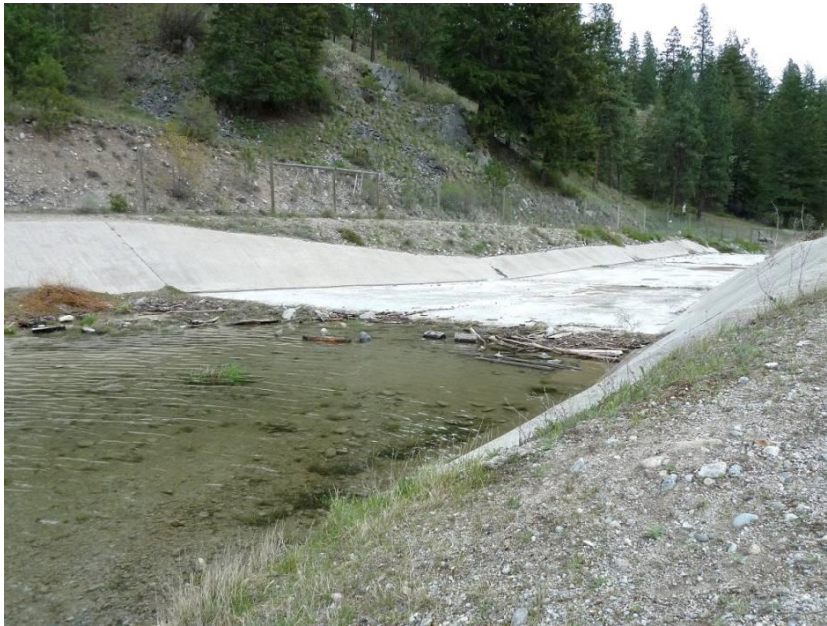
Photo 11.3 Emergency Spillway – Concrete spillway. Some shifting and cracking in concrete. Minor debris. Note road and safety fence.
