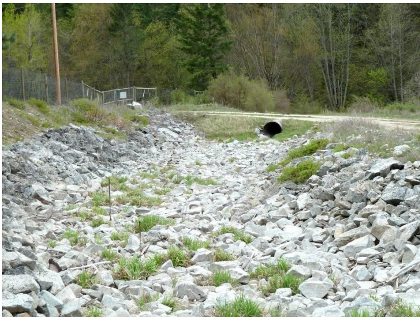
Photo 11.4 Emergency Spillway – Access Road and culvert. Good riprap cover. Culvert and road would likely be destroyed in a major storm event.
