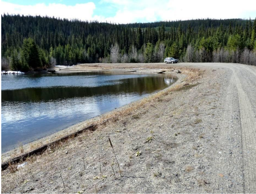
Photo 1.1. U/S Slope of dam – Good condition
