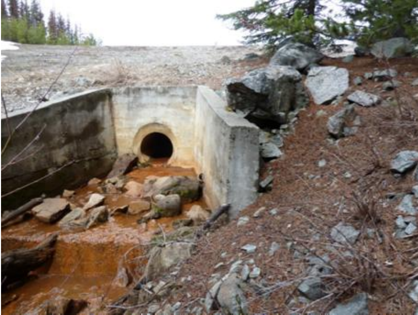
Photo 4.3 Low Level Outlet Structure – Backfill and riprap should be maintained. Rock was plugging outlet at time of inspection. Requires more frequent exercise to clear dirt and debris.
