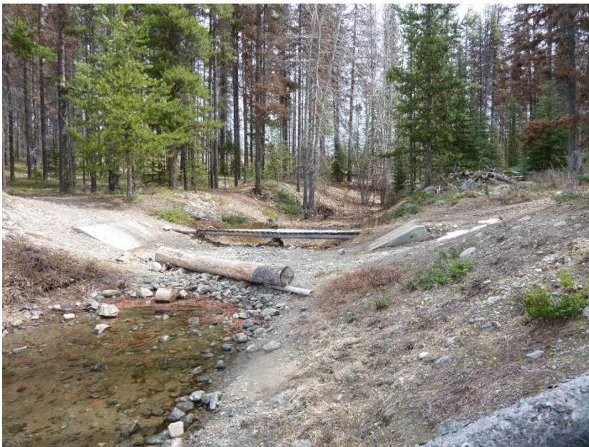
Photo 2.2 Emergency Spillway – Good condition. Requires monitoring for excessive public access and placement of logs and bridges.
