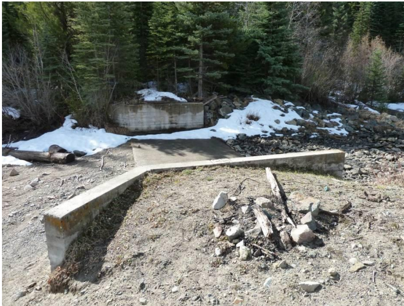
Photo 1.2. Emergency Spillway – Concrete is structurally sound. Note backfill needs and brush removal on far abutment.
