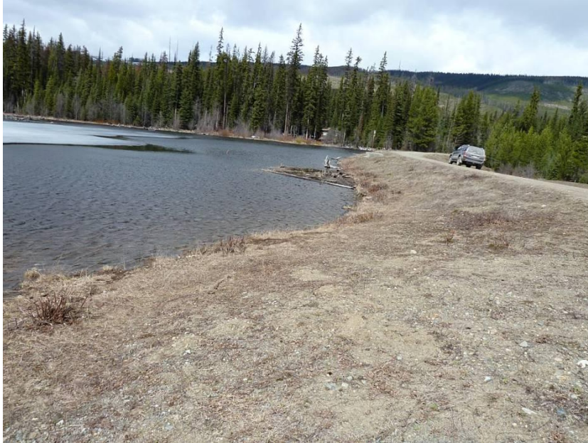
Photo 5.1 U/S Slope of dam – Fair-Good condition. Note old vertical intake pipe.
