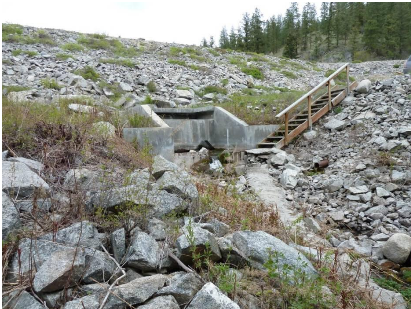
Photo 11.6 Low Level Outlet. Good condition. Seepage flow is from drain outlet beside the structure.
