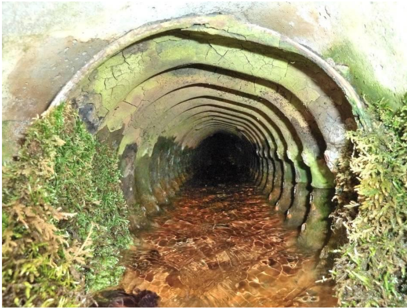
Photo 2.3 Low Level Outlet Structure – Deflection in outlet of CSP pipe. Monitor for further deflections or failure. Requires more frequent exercise to clear dirt and debris.
