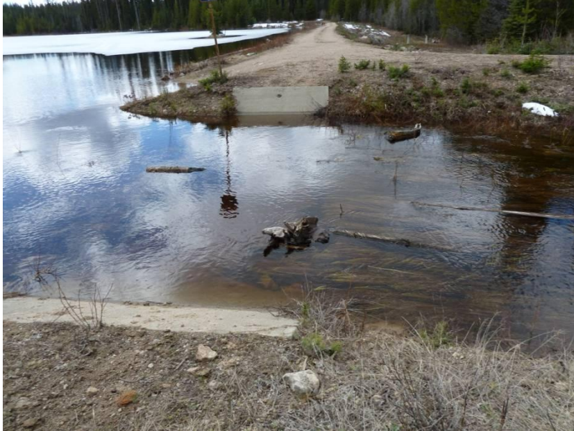
Photo 6.1 Looking across spillway and along center of dam. Water level was at or over FSL at inspection. Difficult to cross to visit dam.
