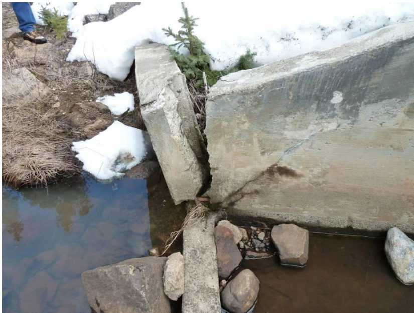
Photo 6.4. General Note: Concrete failure and significant Seepage.
