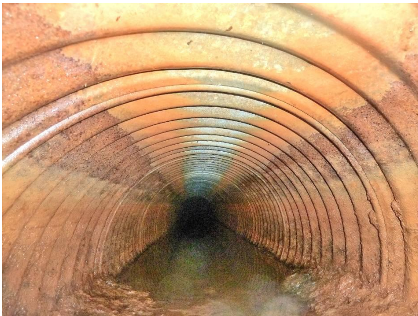
Photo 8.4 Low Level Outlet – Corrugated Steel pipe in fair condition.
