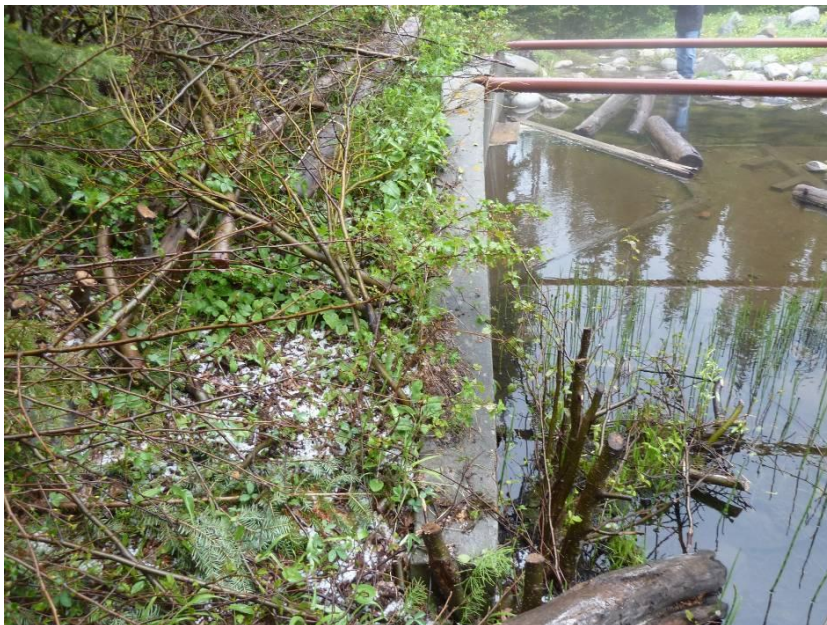
Photo 7.4. Emergency Spillway: Brush intrusion, earth sloughing, excess debris and concrete failures.
