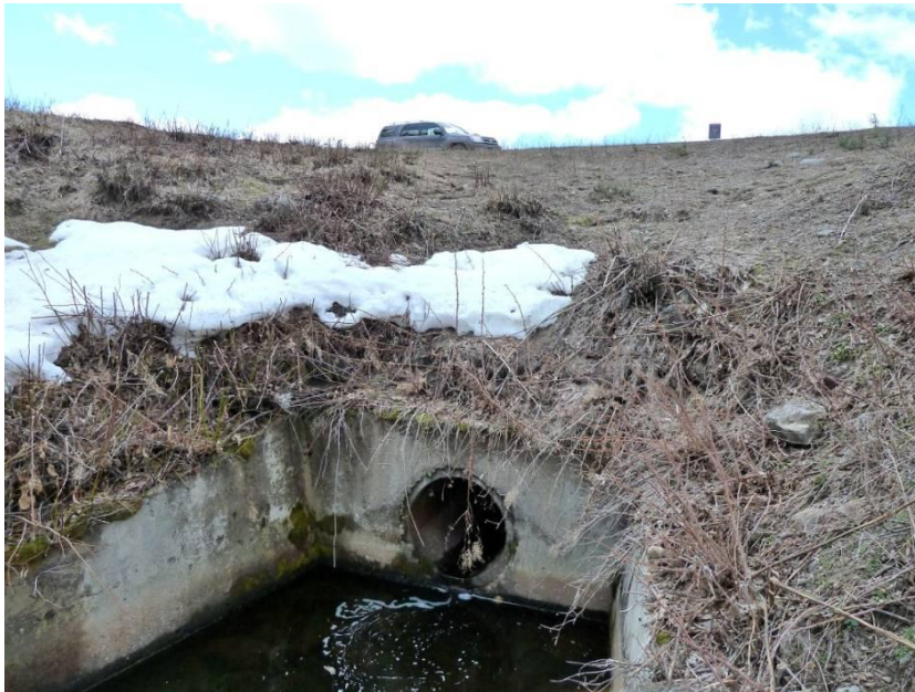
Photo 5.3 Low Level Outlet Structure – Earth backfill is sloughing over the concrete outlet. Brush has been removed. Maintenance required, including additional riprap.
