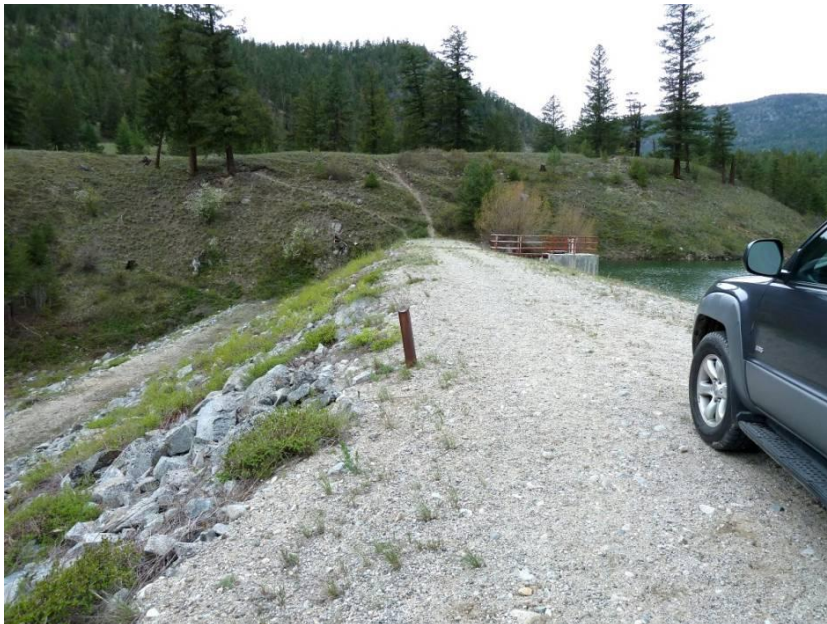
Photo 11.2 D/S Embankment – Steep slope. Riprap is not well defined.
