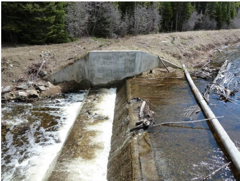
Photo 5.2 Emergency Spillway – Operational. Log boom operational. Required minor cleaning and debris removal.
