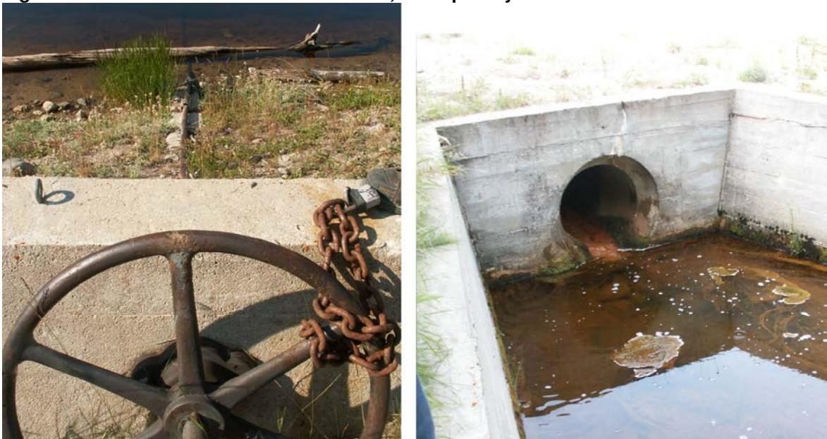
Figure 1.3 – Isintok Gate Control and Outlet, and Spillway
