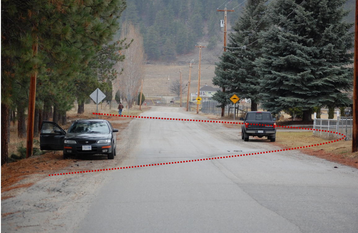
Photograph 3801: Looking west along abrupt roadway depression (dip) that extends across both lanes and to about 5 m into the north property at 10920 Canyon View Road.
