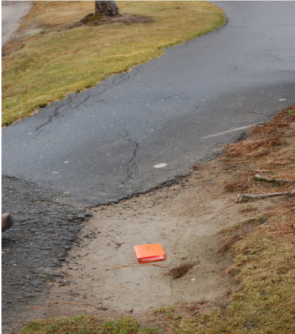
Photograph 3863: Looking south at pavement crack that runs across the golf course pathway and faintly continues across into the ground surface (right hand side of field book) where a 1 to 2 mm wide cracks runs parallel to the slide head scarp that is located about 10 m to the left of the photograph).
