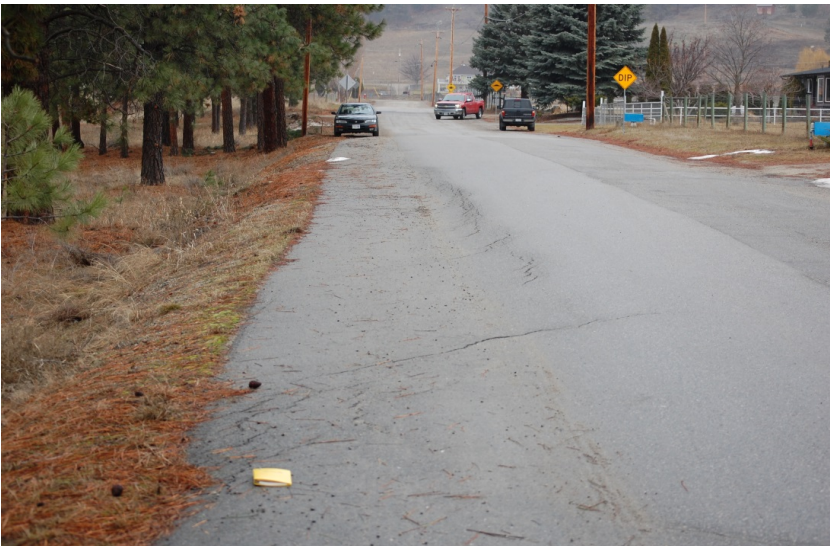
Photograph 3818: Looking west along south outside wheel path with numerous pavement cracks along section of embankment fill that occur in a repeating series having a diagonal pattern.
