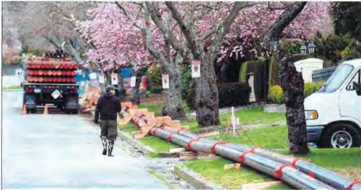
Nearly two million litres of water spill each day from an accidental breach of an aquifer at a house under construction at 7084 Beechwood St. in Vancouver. JASON PAYNE. PNG / VANCOUVER SUN
