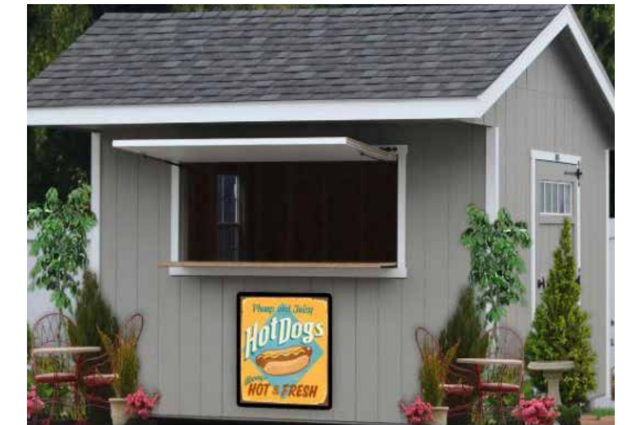
NEW CONCESSION BUILDING
