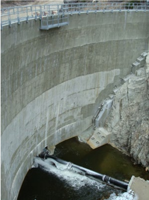
The District's Thirsk Reservoir Dam
