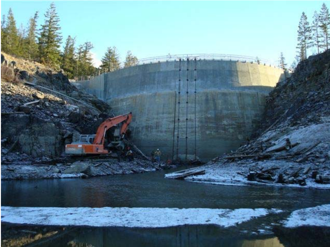
Thirsk Dam on Trout Creek - Upstream Face
