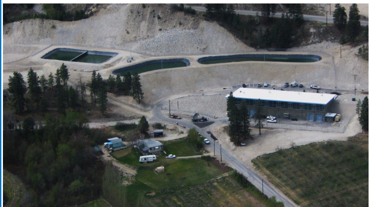
Summerland Water Treatment Plant
