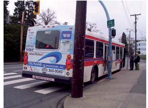
Crosswalk located too close to stop, (contravenes Motor Vehicle Act) utility pole blocks exit door and driver sightlines. Utility pole blocking pedestrian curb cut.
