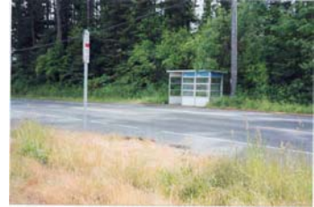
At night these stops no longer feel safe: they are isolated, landscaping is overgrown creating "hiding spots" and there is no lighting nor any houses looking on.
