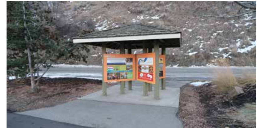
Image of the existing information kiosk at Peach Orchard Beach Park.
