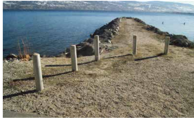
Breakwater and bollards
