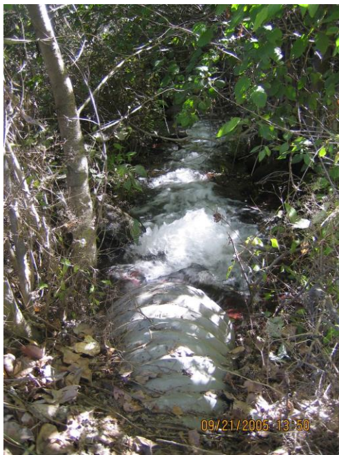
South Side – Looking South
