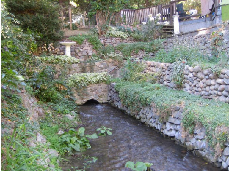
South Side – Looking South
