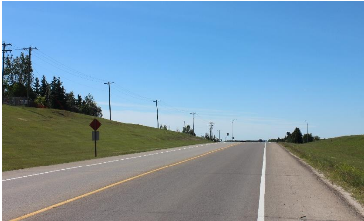
Figure 21. Bicycle Accessible Shoulder
