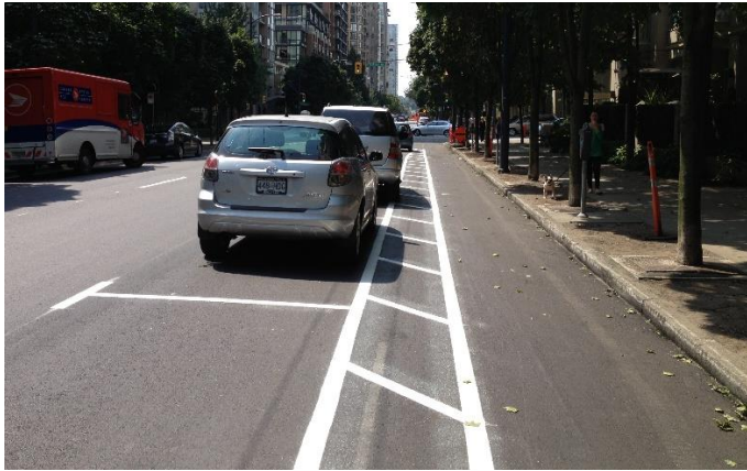
Figure 16. Buffered Bicycle lane
