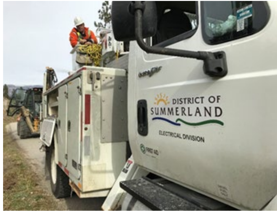
Electrical Division vehicle. Source: District of Summerland
