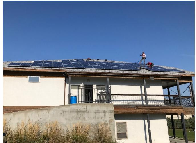
17.25 kW solar PV array being installed on Arts & Cultural Centre
