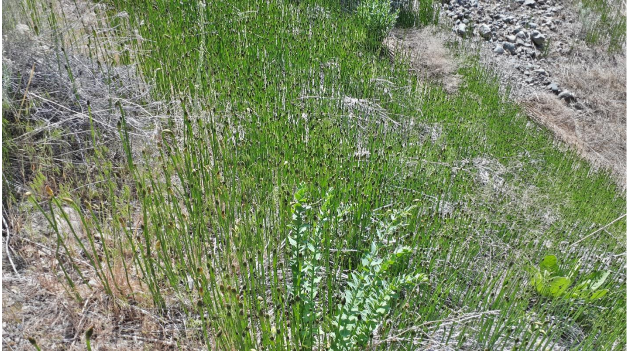
Photo Four. Seepage from excavation cut has allowed horsetail to establish. Wetland noted is just off frame to the right.
