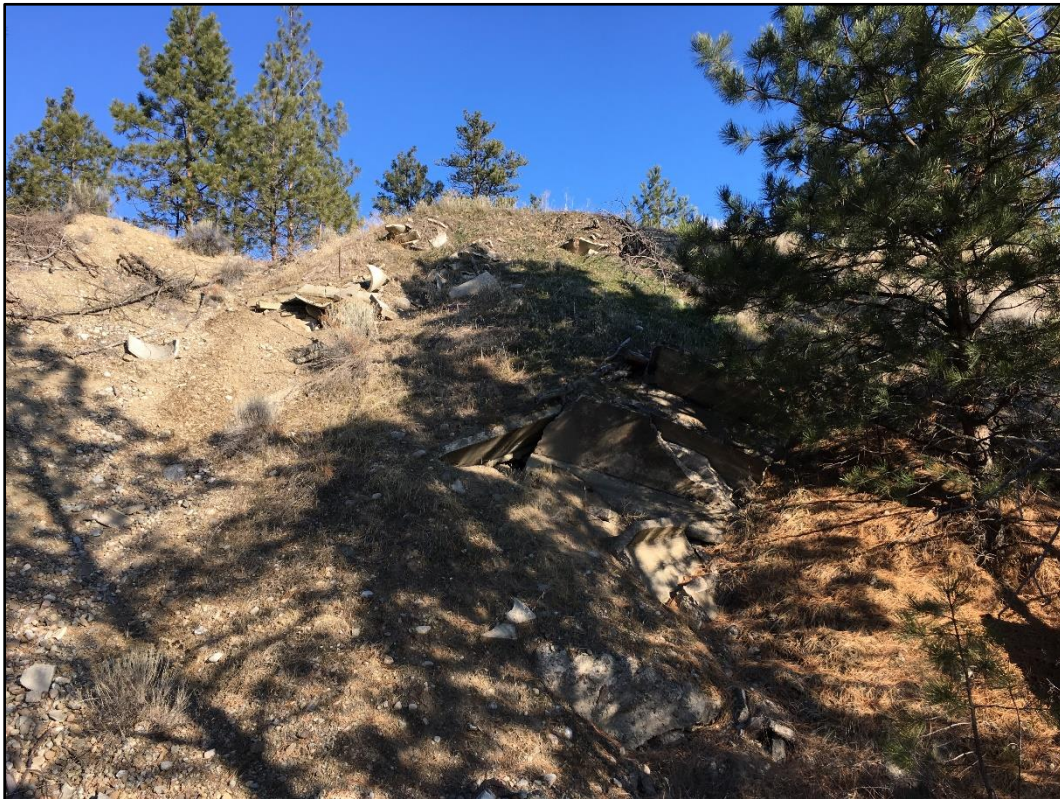
Photograph 8: View of concrete debris located North of APEC #4 (November 29, 2019).
